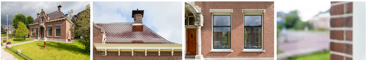
Figure 2. Case in Leens after the construction process (Mark Sekuur, 2024).
