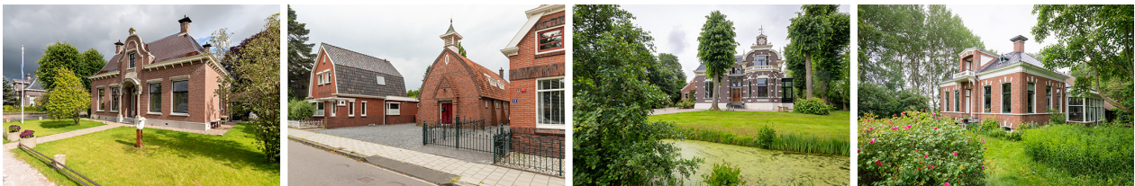
Figure 1. The case study buildings: Leens, Musselkanaal, Appingedam, and Spijk (Mark Sekuur, 2024).
