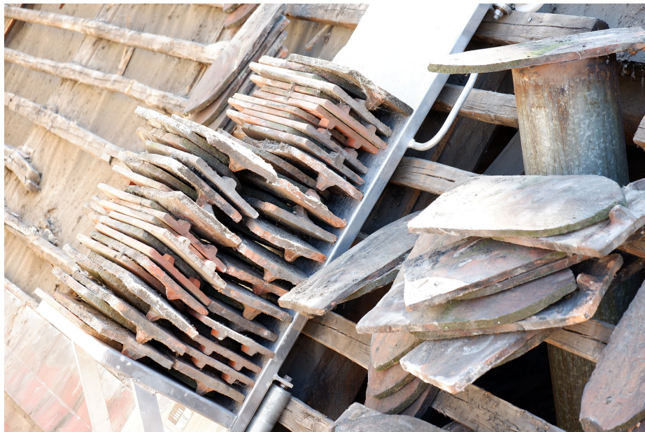
Figure 3. Salvaged tiles stacked on the roof of Georgenstraße 53b, Amberg, ready to be transported into storage (2023). Source: Courtesy of Jana Scher.
