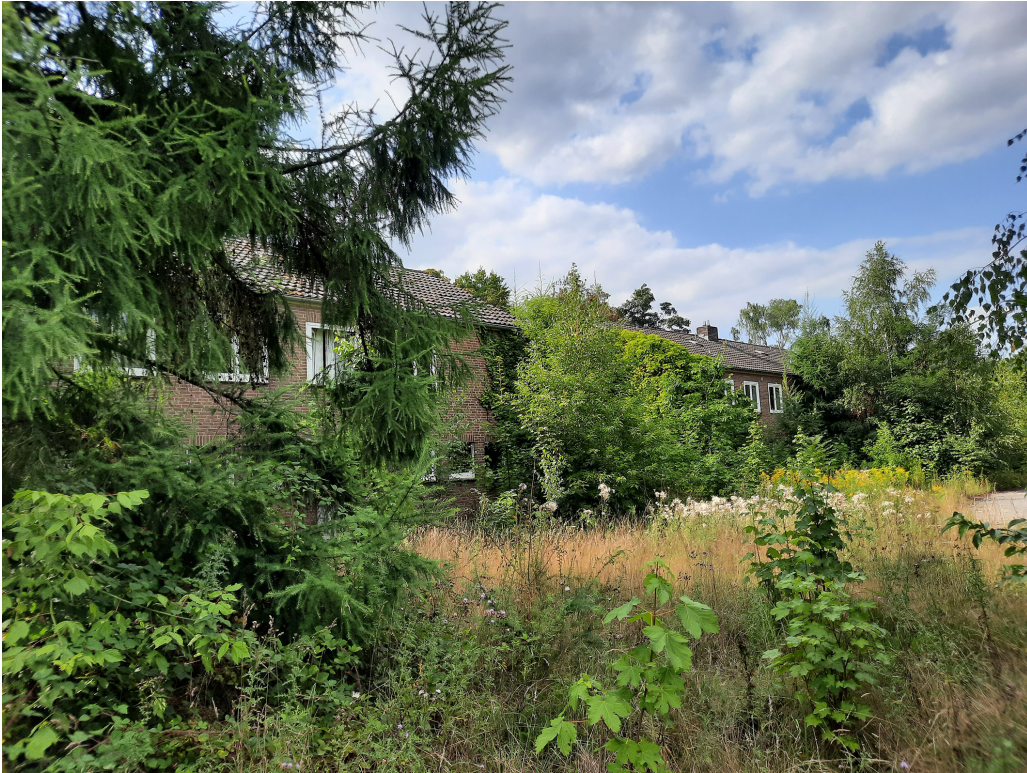
Figure 2. Interior of JHQ Rheindahlen, showing decaying structures.
