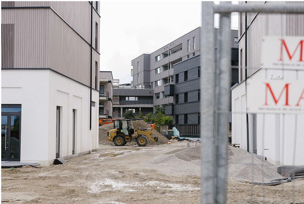
Figure 5. Building site Munich-Freiham in summer 2025. Photo by Johanna Niesen.
