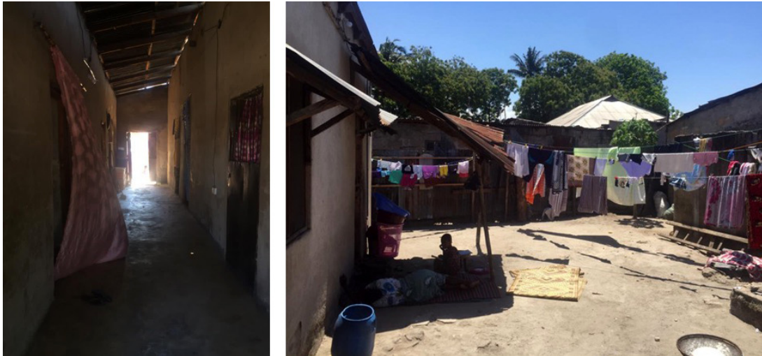
Figure 4. Core elements of the Swahili house: The central corridor provides structure, connectivity, and thermal comfort; the courtyard offers privacy in an open space, in contrast to the public front veranda. Source: Courtesy of Beatrice Mahagama and Leticia George.
