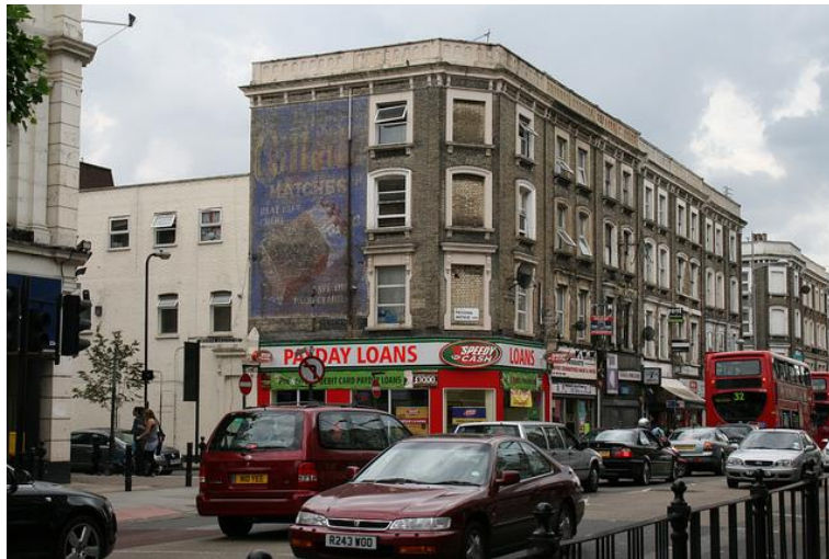
Figure 4. A panorama of KHR shopfronts. Source: Flickr, The Creative Commons.
